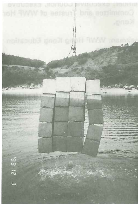
Strings of twenty reef blocks are lowered into the sea at Hoi Ha Wan.
